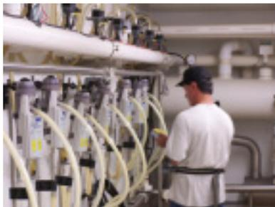
When using these meters in a basement parlor we listen for side to be released then go down the whole side and press finished milking buttons. This parlor we have a problem where the equipment dealer did not mount one pipe tight and it keeps turning on us. These meters will compensate for being a bit out of level.
